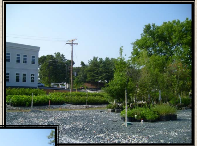
Staging area with material for projects
